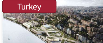
Galataport İstanbul Project - Salıpazarı and Package Post Office İstanbul Modern Art Museum
